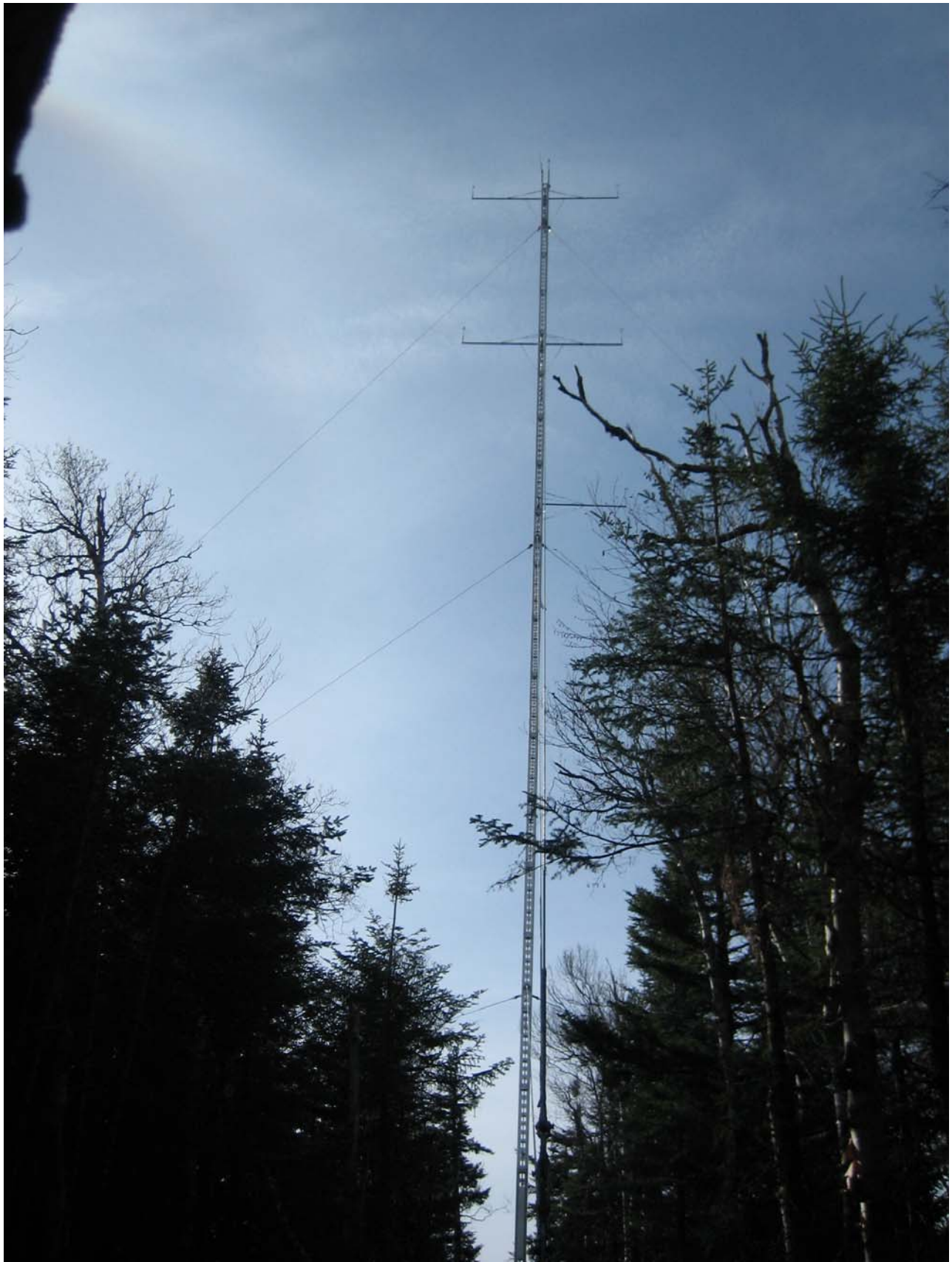
Figure 2-21. Existing Met Tower
