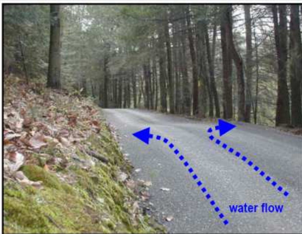
GRADE BREAK – Interruption in slope redirects flow and causes water to leave road area.
